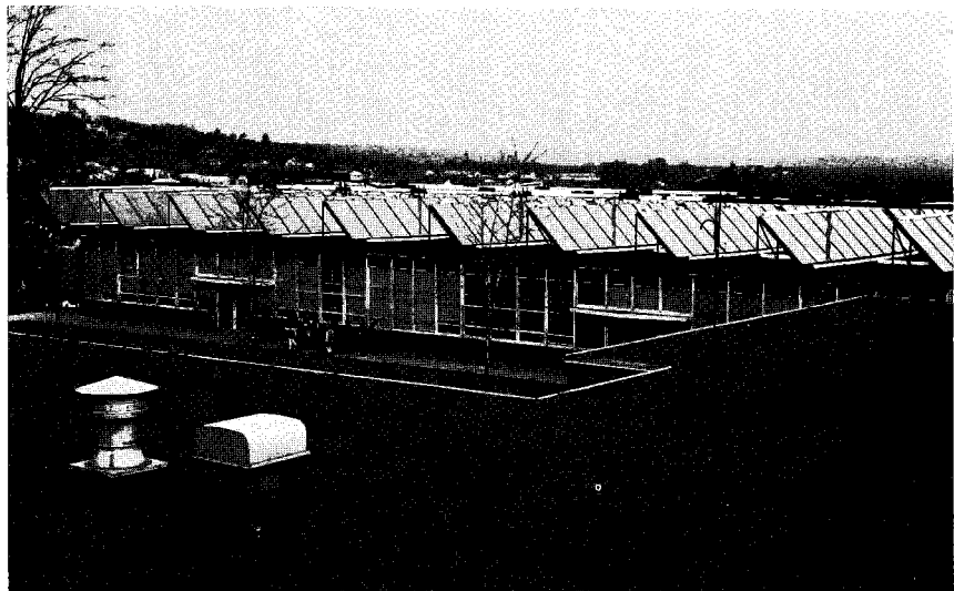
The Timonium Elementary School near Baltimore, Maryland, one of four schools that experimented with NSF-sponsored solar heating systems last year, was the first school in the Nation heated by solar energy. Solar heat is collected in water flowing through the rooftop panels, pumped into a storage tank, and then used to heat classrooms. [Photo by Aircraft Armaments, Inc.]
