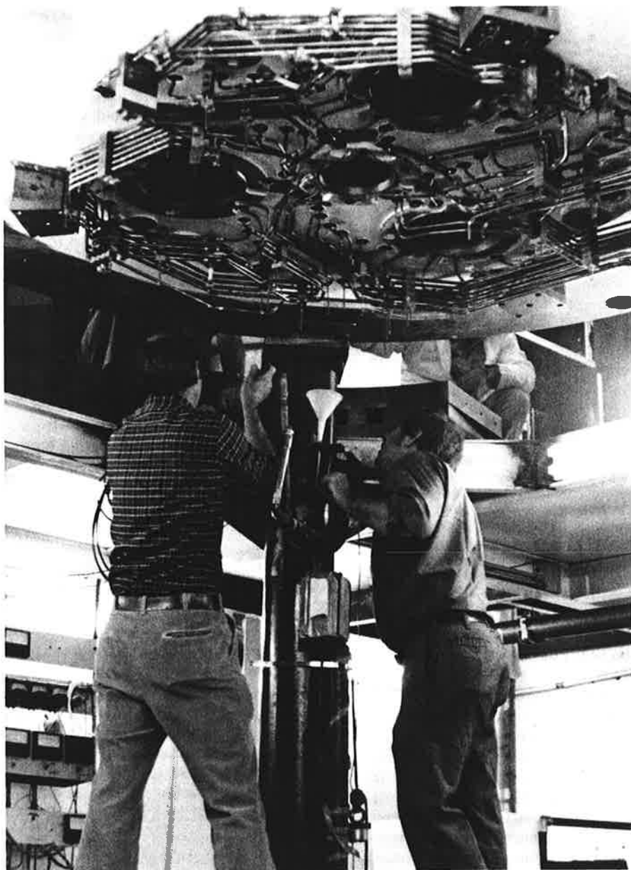
Studies of nuclei. At Michigan State University's Superconducting Cyclotron Laboratory, workers install the bottom cap of a cyclotron magnet. The copper piping on the cap feeds current and water to coils elsewhere in the magnet. This accelerator for heavy ions is an important tool in nuclear physics research and experimentation.
