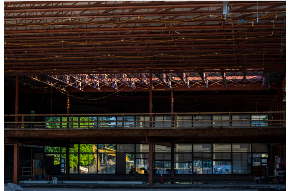
Rehab Hewitt Hall - Phase I
