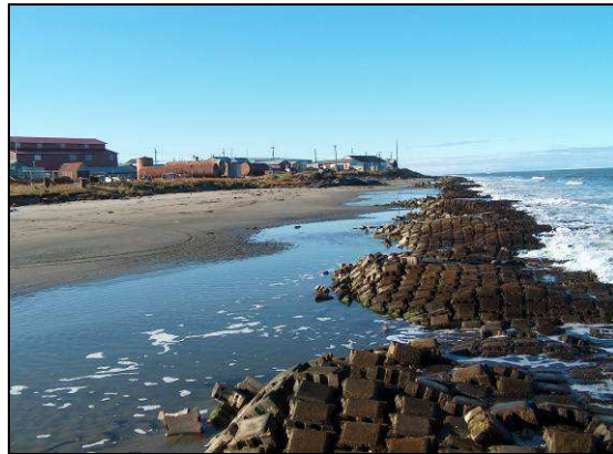
Old articulated concrete mat project
