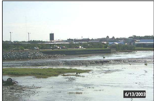
Corps protection on harbor east bank
