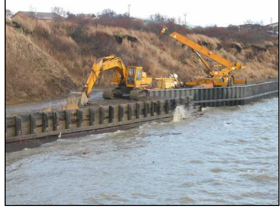
Corps shore protection at Snag Point
