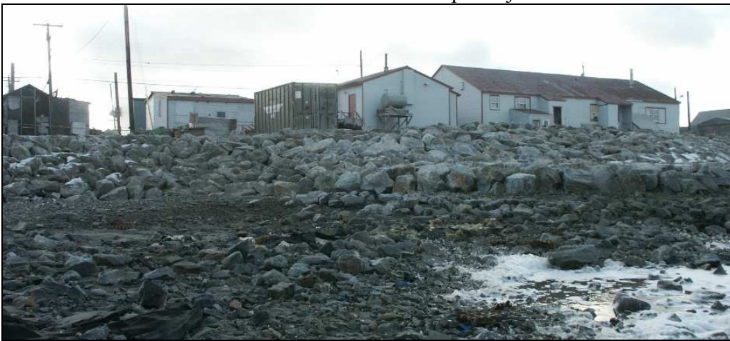
Post Construction – Corps Project to Right / City Project to Left in 2005
