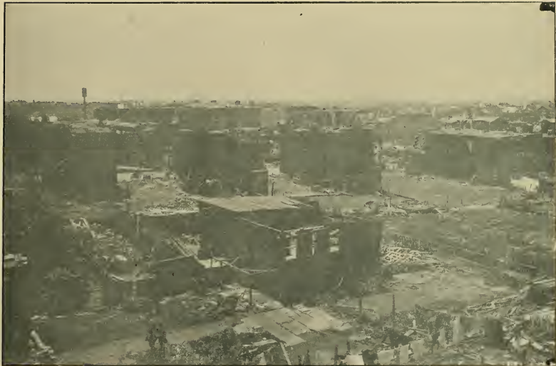
LOOKING SOUTHWEST FROM MISSISSIPPI AND LAFAYETTE AVENUES
