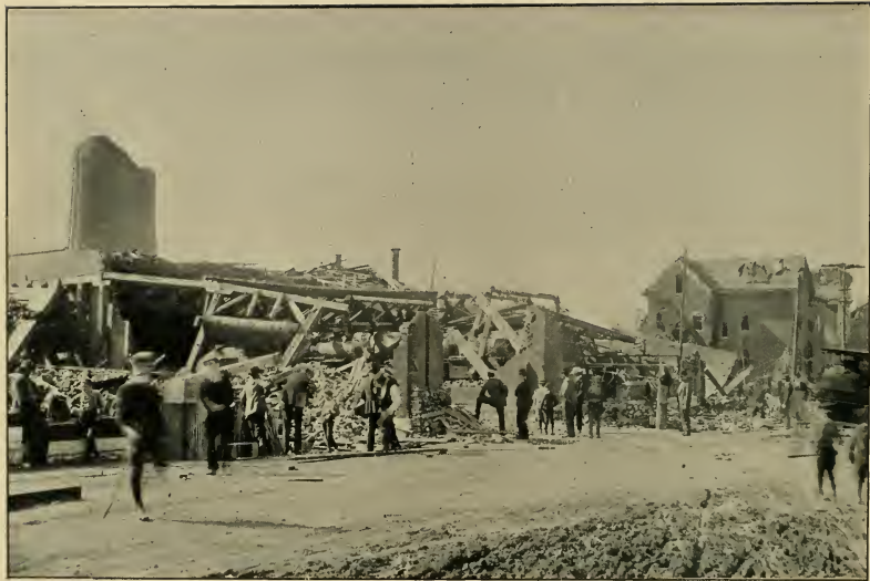
RUINS AT GEYER AND JEFFERSON AVENUES
