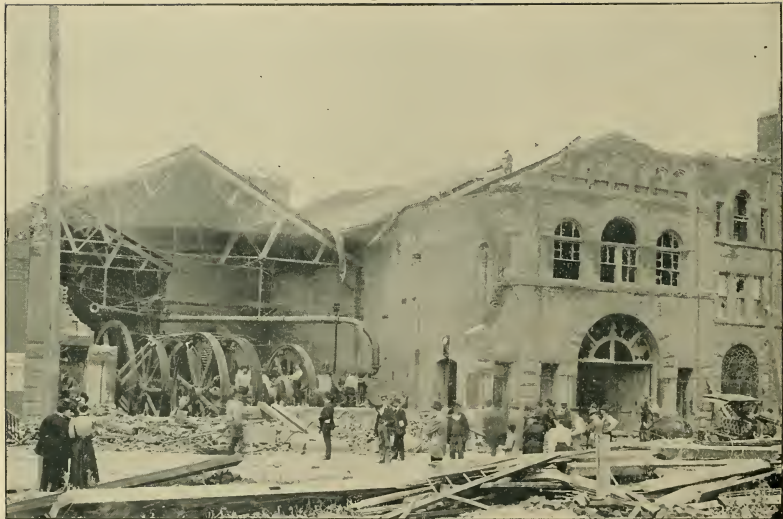
PEOPLE'S RAILWAY CO.'S POWER HOUSE
