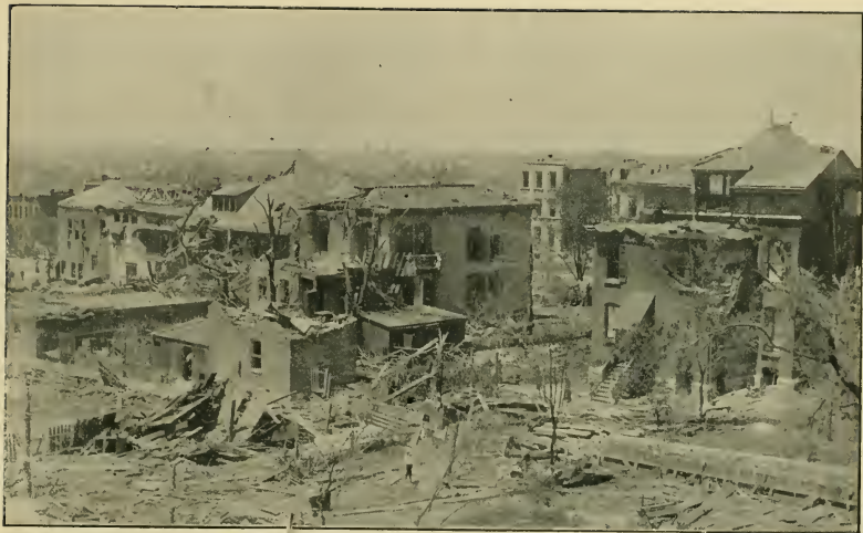
WRECKED RESIDENCES IN THE LAFAYETTE PARK DISTRICT
