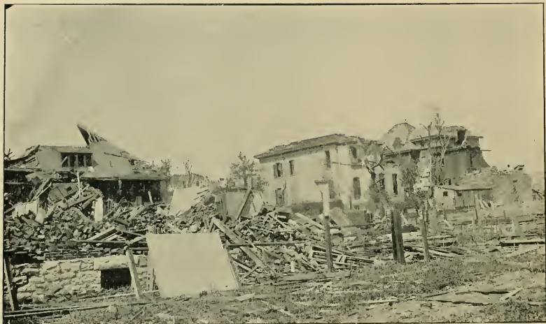
WRECKED RESIDENCES IN THE LAFAYETTE PARK DISTRICT
