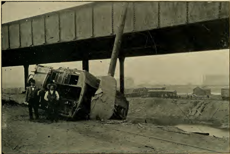
ELECTRIC CAR BLOWN FROM THE EADS' BRIDGE
