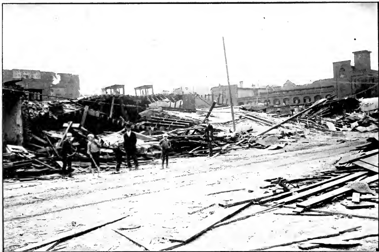
WAREHOUSE ON TWELFTH AND GRATIOT STREETS
