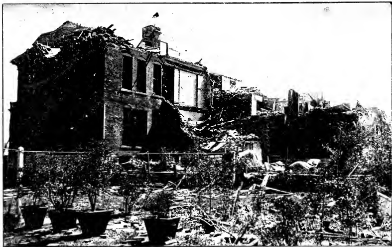
WRECKED RESIDENCES IN THE LAFAYETTE PARK DISTRICT
