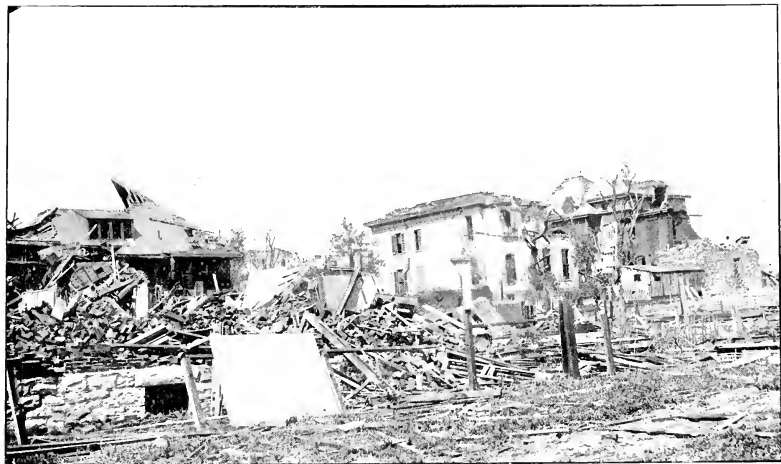
WRECKED RESIDENCES IN THE LAFAYETTE PARK DISTRICT
