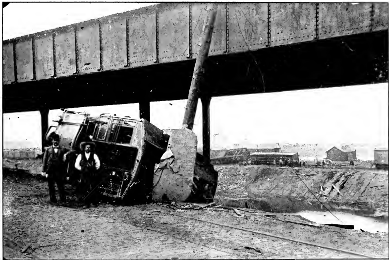
ELECTRIC CAR BLOWN FROM THE EADS' BRIDGE
