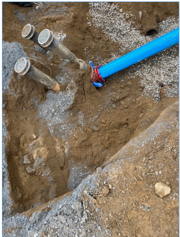
New PVC Water Main
