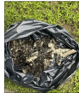
Fats Oils & Grease Being Removed and Disposed of Before Clogging the Sewer Field
