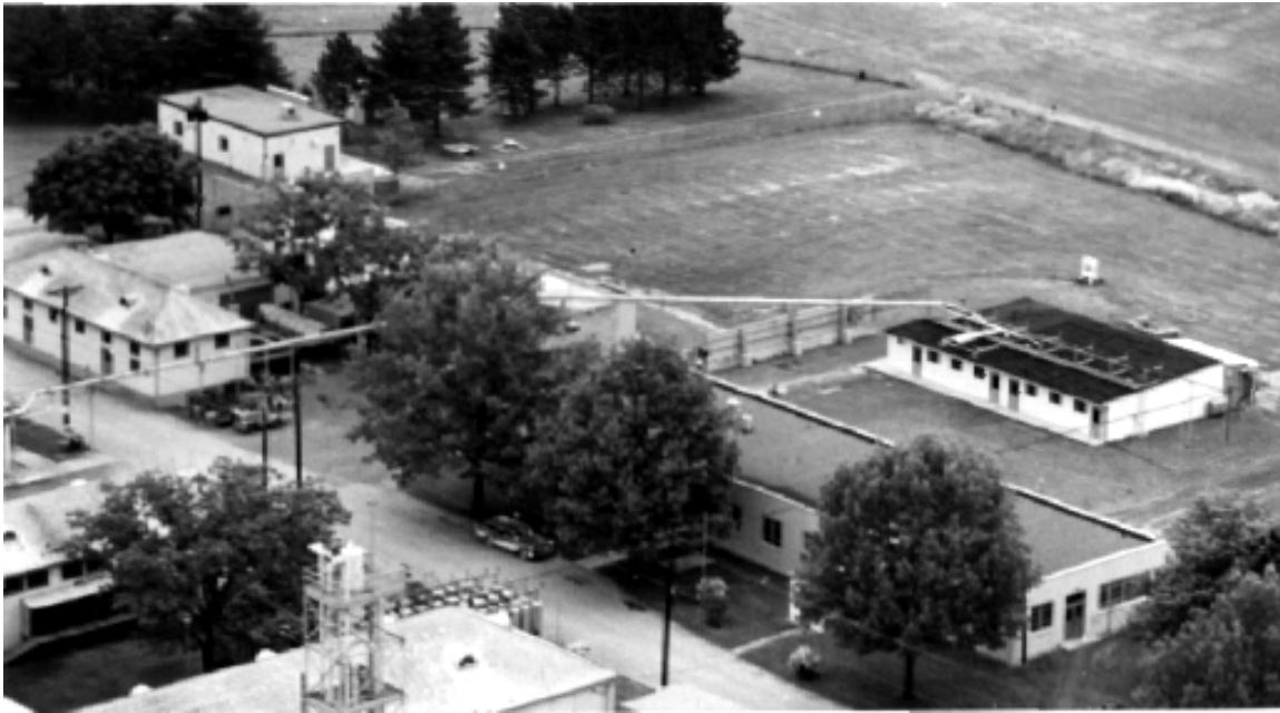
Figure 15: View of Forrester Campus facilities. The office building is in the center of the photograph with experimental areas behind it. To its rear are the atmospheric test facilities and to its left, partially obscured, are the liquid propellant rocket test cells. The bottle farm and ejector tower servicing the supersonic and hypersonic facilities may be seen in the lower left. The solid propellant processing laboratory is in the upper left hand corner. June 1962.
