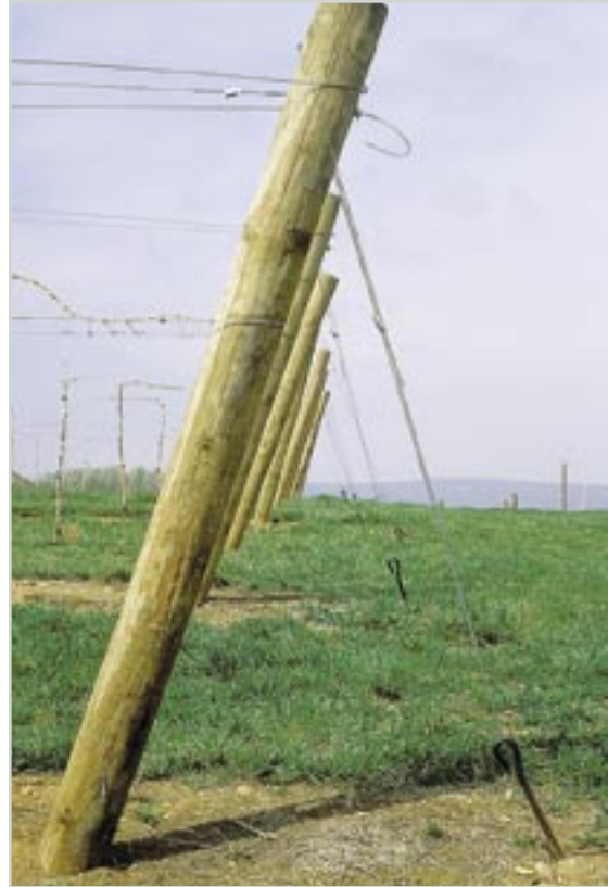
FIGURE 23. End posts are set 3 feet in the ground at a 60-degree angle and anchored with a screw-type steel anchor.
