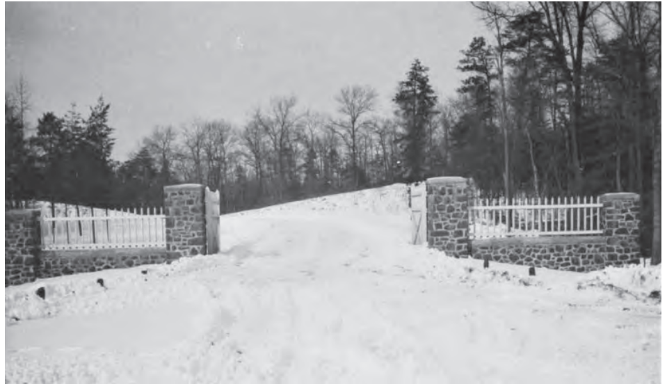
Stone gate built by the CCC camp and metal white picket gate and fence built by WPA shop, winter 1938-39.
