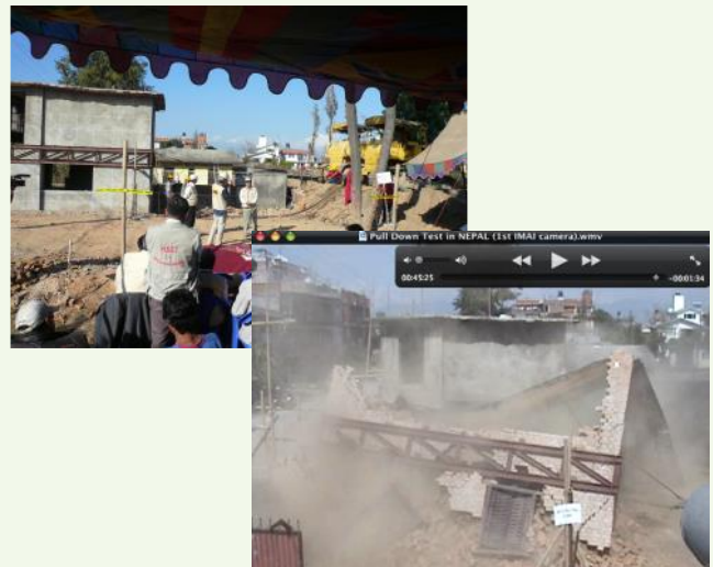
Figure 2-40 Pull-Down Test for Seismic Resistance of Building
