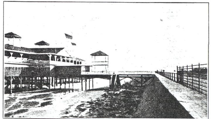
FIG. 3.—Sea wall and pavilion at Galveston, Tex. The riprap at the bottom and the curved face of the wall break the force of the waves. The pavilion was destroyed by the storm of July 21, 1909.
