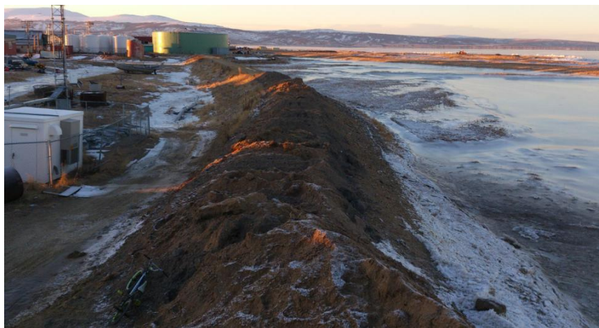
Figure 10. Temporary levee project from fall 2013 (photo by Carol Oliver, 2013).
