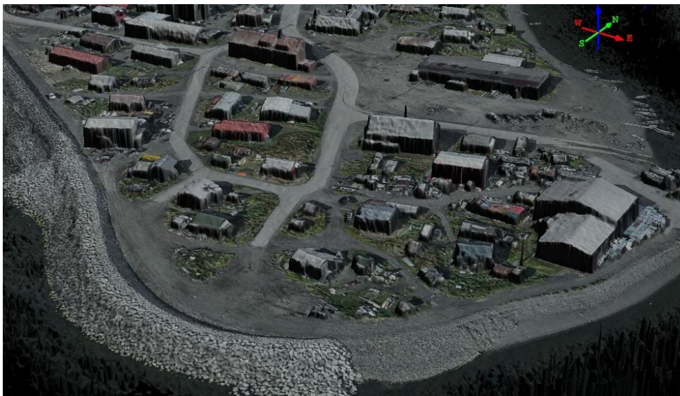
Figure 8. 3-dimensional model view of the Unalakleet revetment looking north from the inlet. (2014 aerial image draped over DEM provided by Fairbanks Fodar, 2014).
