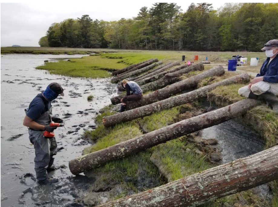
Living shoreline installation in Brunswick, ME. Image credit: P. Slovinsky, Maine Geological Survey.
