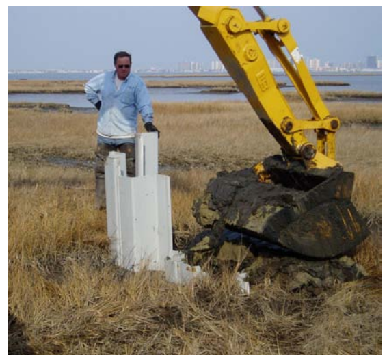
Insertion of the polymer sheets to form a ditch plug / Kevin Smith, MD DNR Watershed Services
