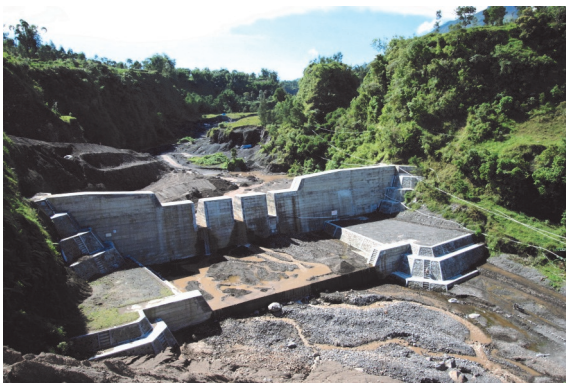
Erosion control facility using Japanese technology (Indonesia) Photo: JICA
