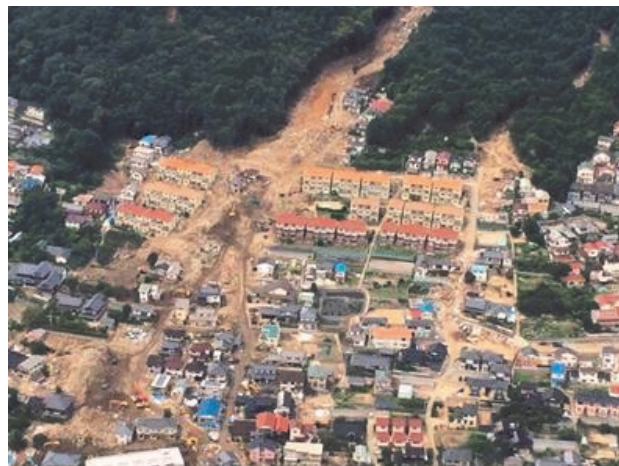
View of the sediment disaster in Hiroshima
