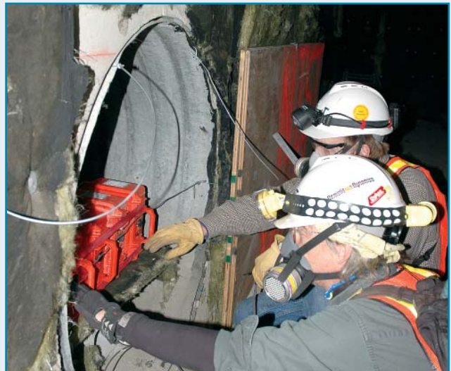
NIST electrical engineers Chris Holloway and Galen Koepke place transmitters in a protected air vent at the old Washington Convention Center prior to the implosion of the building. The experiments were performed to help improve the communication capabilities for emergency first responders.
