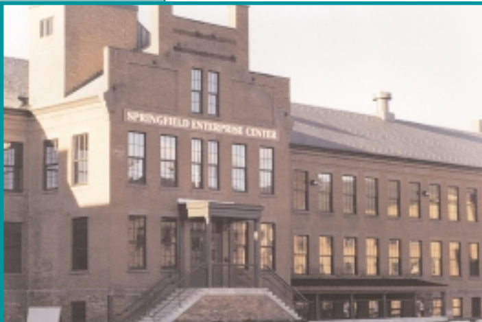
Springfield Technical Community College (STCC) constructed Springfield, Massachusetts' first facility dedicated exclusively to the launching of the new high tech business initiatives and assisting recent start-ups achieve profitability with the assistance from an EDA project. The incubator is located in the center of Springfield's two major disadvantaged areas where poverty and unemployment are the highest in the area.
