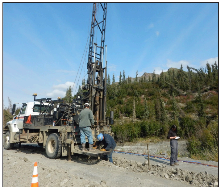
DOT&PF crew drilling test hole at FDL-A site, August 2020.
