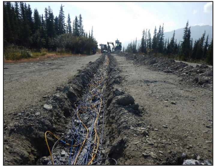
Trench with geomechanical instrumentation wires to ADAS.
