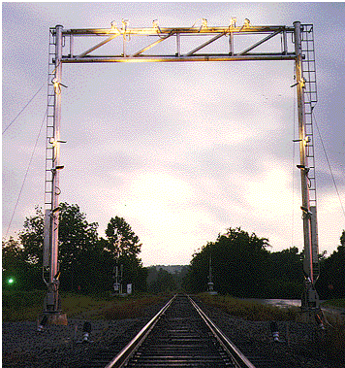
Figure B.2. Car Clearance Detection System
