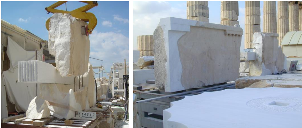
Figure 2. Joining together the ancient fragments \epsilon and \zeta (see Fig.1) and new supplements (on the left). The aforementioned complex is joined to the rest, already restored, eastern part (on the right).
