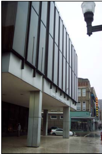
The former United Way building on Broad
