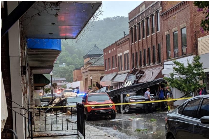
A portion of the roof of the Hock Shop on West Court Street
