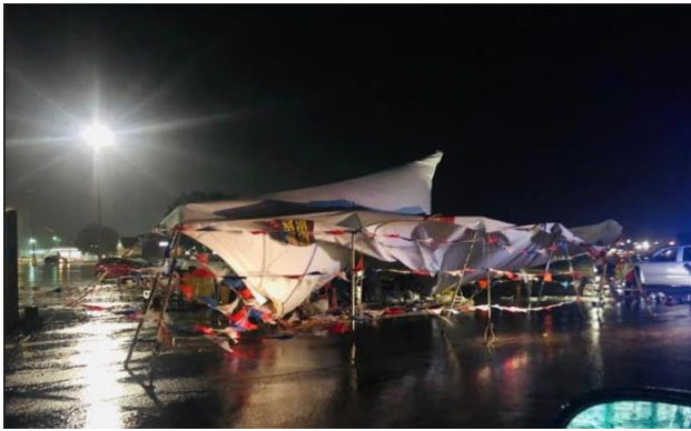
June 21 st collapsed firework tent in Monticello Courtesy of WYMT
