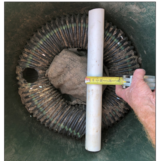
Figure 2. Fill tube cut to length with a 30-degree angle cut on one end.
