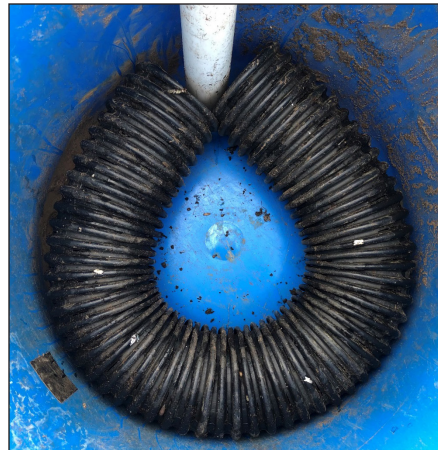
Figure 4. Butting the ends of the perforated pipe creates a void for installing the fill tube.
