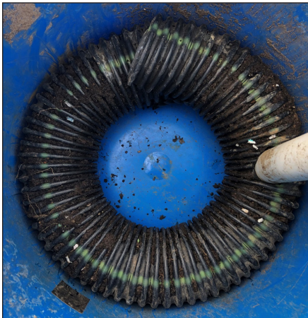
Figure 3. Perforated pipe overlapping itself. Fill tube hole installed using a hole saw.
