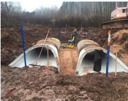
Culvert replacement. Photo courtesy of Eric Andrews.
