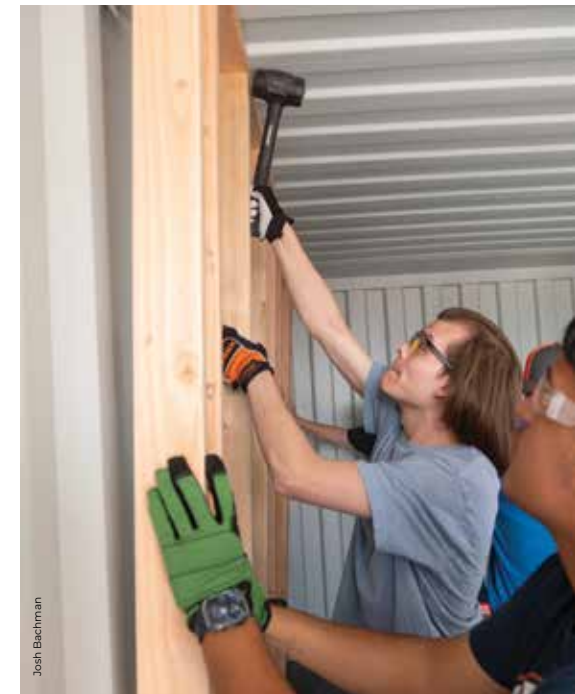
Doña Ana Community College students build and install an interior frame for a 20-foot container farm that will be housed on NMSU’s Las Cruces campus. The Las Cruces container farm is a collaboration between the College of ACES, College of Engineering, DACC and NMSU’s Center of Excellence in Sustainable Food and Agricultural Systems.
