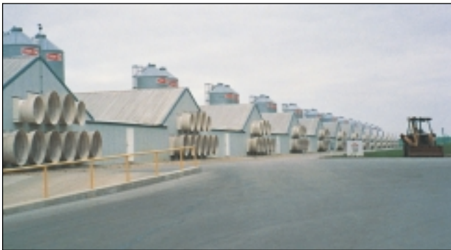
Figure 1. Typical environmentally controlled layer house. (00-CN-0601)
