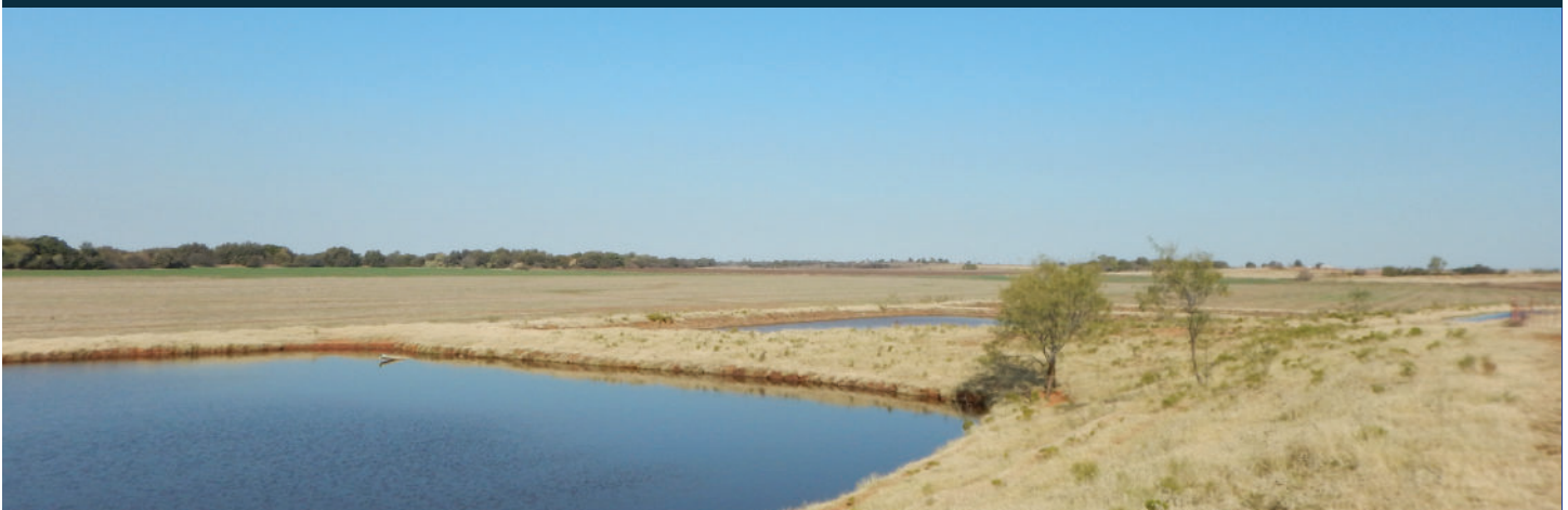
Photo 8: This facility's lagoons are designed, constructed, operated and maintained to contain all process-generated waste and process wastewater plus runoff from a 25-year, 24-hour rain event.
