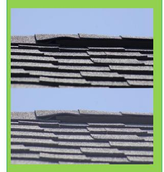
Top photo: Ridge vent before illumination: Bottom photo: Ridge vent after illumination. Note how the hole, which can allow bat entry becomes visible.
