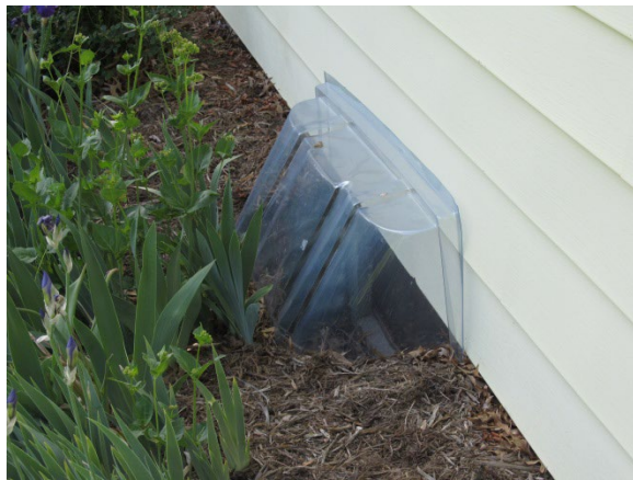
Figure 6. A plastic window well cover.
