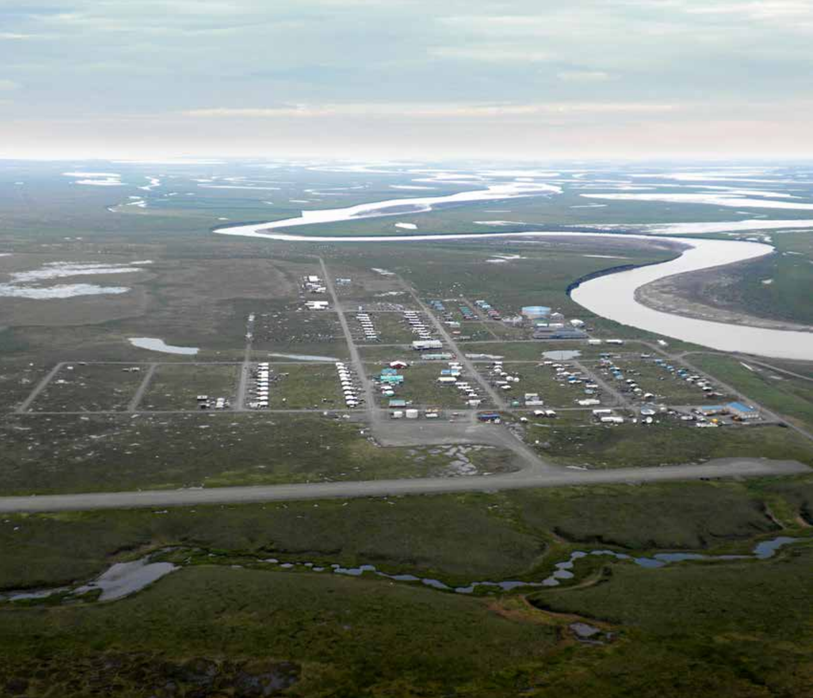
Aerial view of Nuiqsut. Mike Brubaker, 2013.
