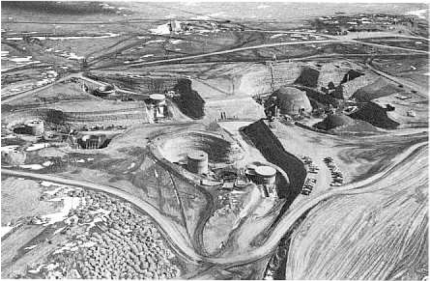
Titan missile Site 1A, under construction at Lowry AFB, Colorado, February 1960.
