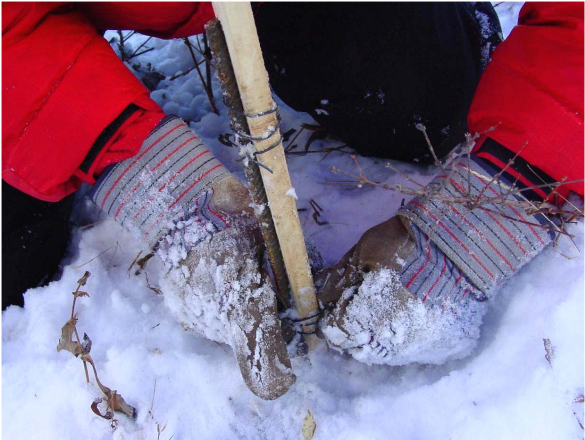
Figure 8. Attaching wooden posts to rebar in October, 2004.
