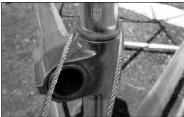
Figure 7. A simple guy wire connection to leg above the upper cross arm. Note the double wrap around the tower leg.
