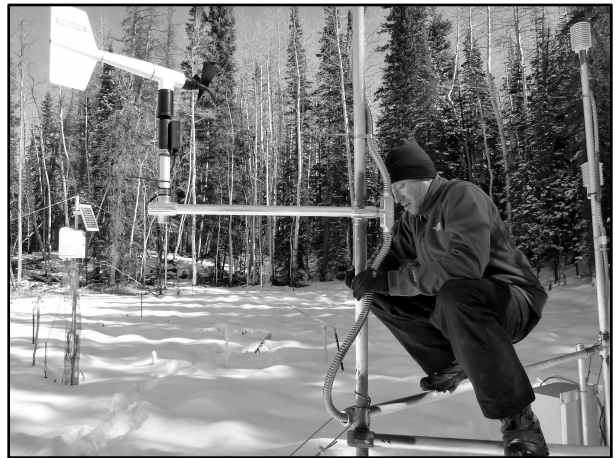
Figure 11. Daniel Bowker tightens hose clamps above and below a cross arm to secure flexible conduit. Wires were combined in all possible runs to reduce the number of individual conduits and connectors, as well as the number of ports into logger and battery boxes.
