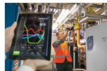
BUILDING AUTOMATION SYSTEMS
