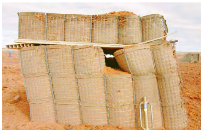
Figure 2. Heavily damaged but stable structure
