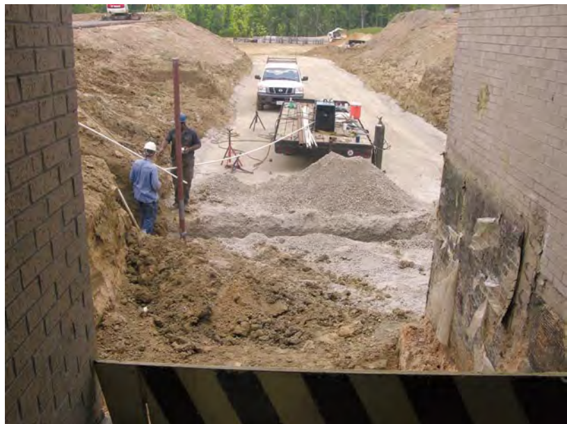
Utility corridor begins to take shape
