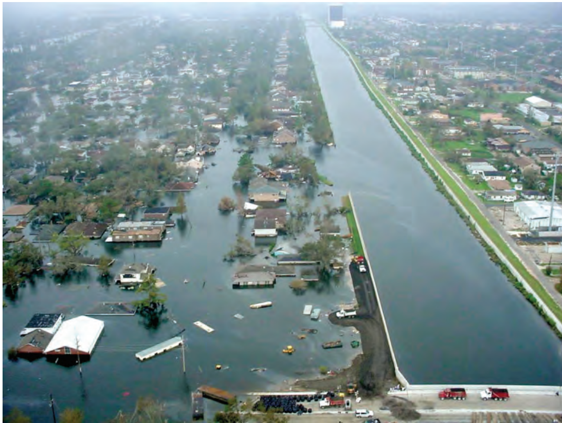
The IPET Risk and Reliability analysis will give the decision makers information on how the hurricane protection system will perform after repairs are completed on the Katrina-damaged sections on June 1, 2006
