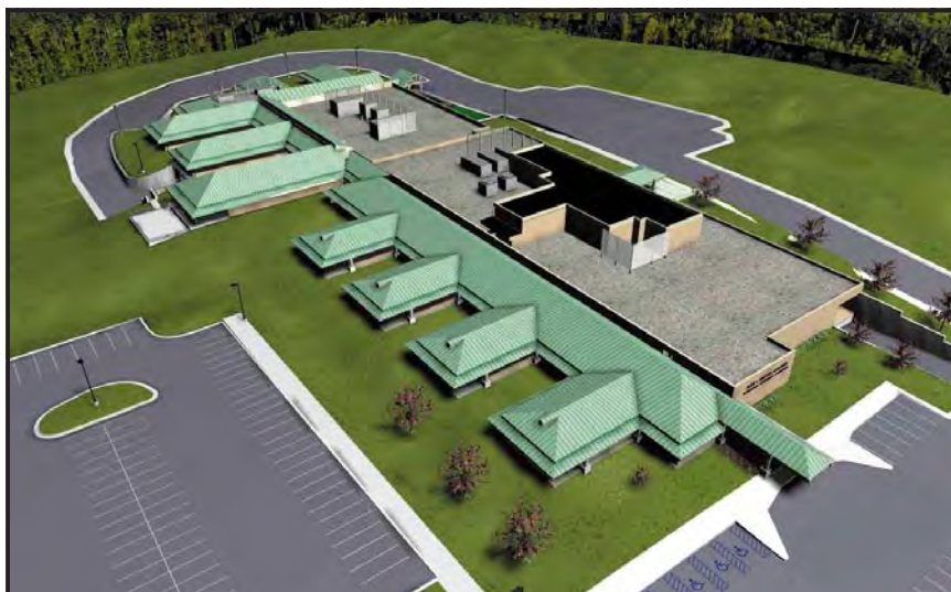
The Jamie L. Whitten building, headquarters of the Information Technology Laboratory founded by Dr. N. Radhakrishnan
