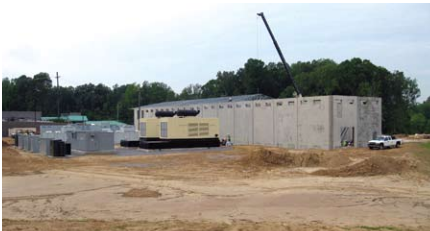
Construction site on April 29, 2009
