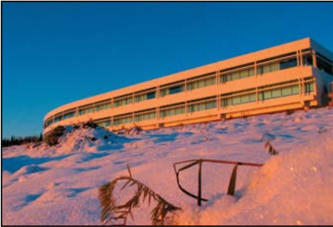
The Butrovich Building on the University of Alaska campus in Fairbanks as seen on a crisp, clear late autumn day. ARSC supercomputers and storage facilities are located on the lower floor of the building
