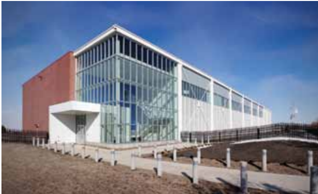
The 88,000-square-foot National Petascale Computing Facility in Champaign, IL, includes a 20,000-square-foot data center with an additional 10,000 square feet of raised floor for other infrastructure
