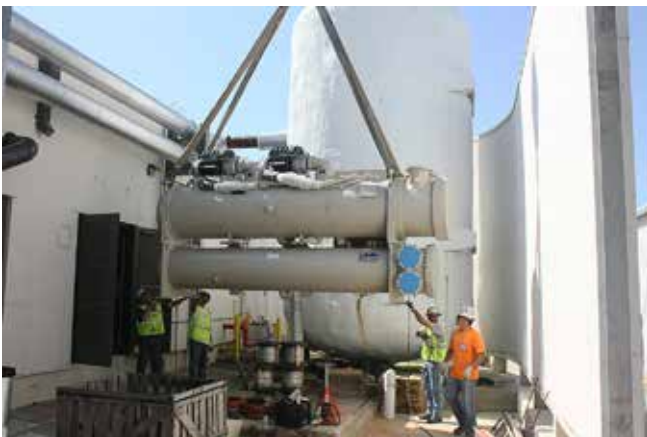
The 300 ton chiller's eventual location is just inside the double doors on the left of the picture. The chiller had about 1/2" of clearance going through the doors.
