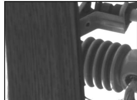
Figure 4C. Image of power transformer taken with parasol.
