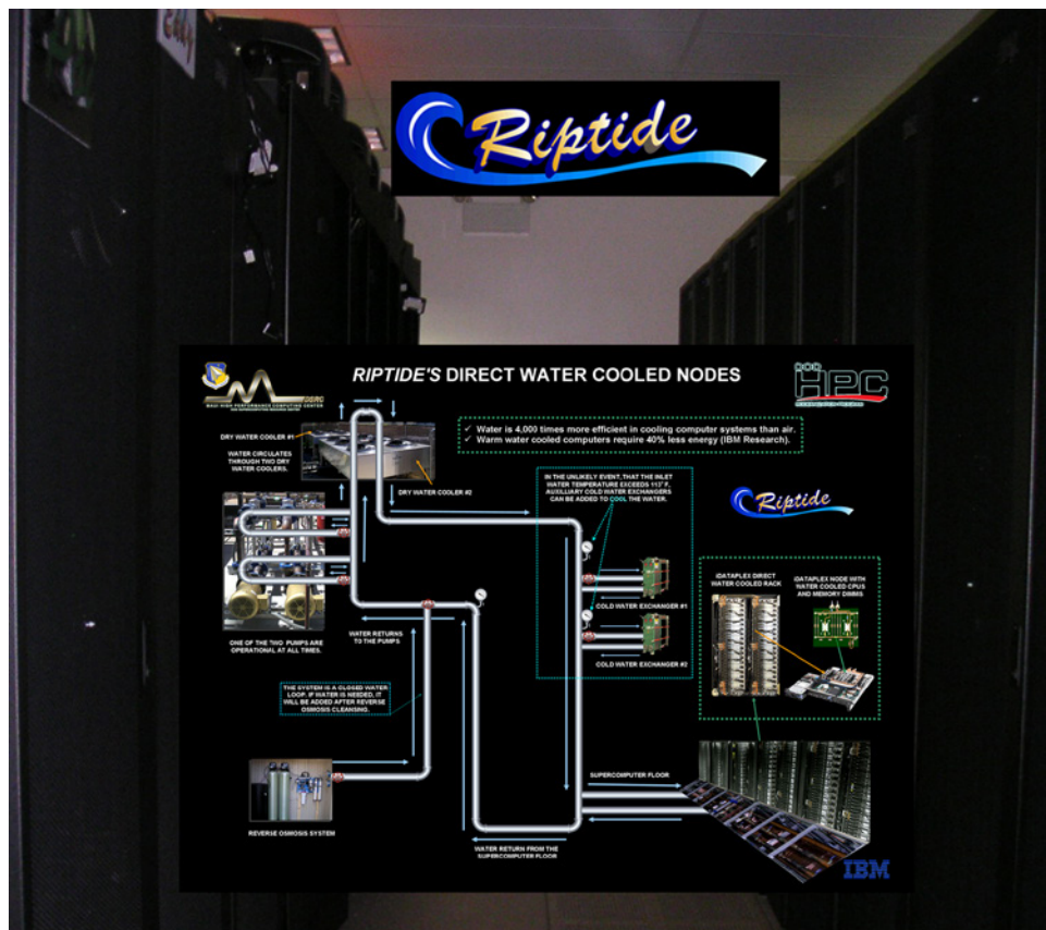
IBM iDataPlex ( Riptide ), MHPCC DSRC
