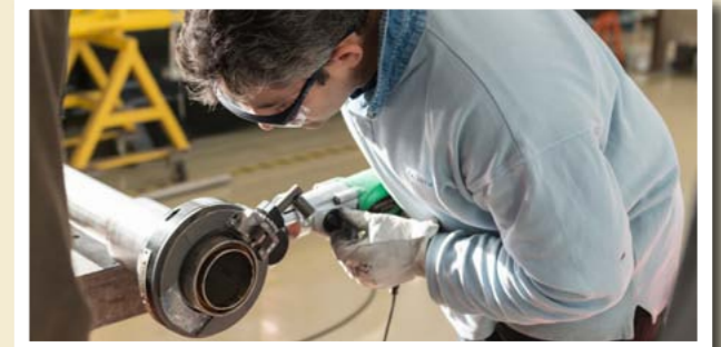
The cutting tool used to open the busbar lines.
