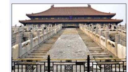
Workers probably slid massive stones, such as this 300 tonne marble carving in front of the Hall of Supreme Harmony in the Forbidden City, along artificial ice paths.
