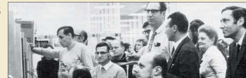
In the ISR control room.
