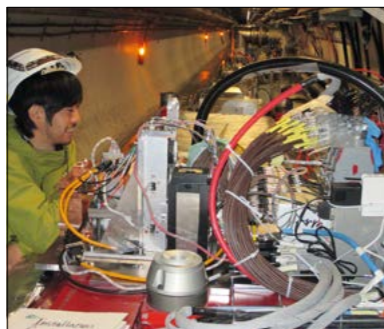
LHCf's Arm1 detectors installed in the LHC tunnel. (Image credit: T Sako.)
