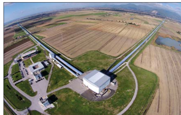
Virgo, located near Pisa in Italy, has arms that are 3 km long and was the first detector in Europe – and the third ever – to register a passing gravitational wave.
