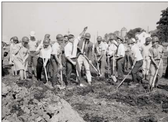
Ground-breaking for the 200 GeV Synchrotron/Main Ring at the National Accelerator Laboratory in October 1969.
