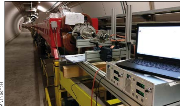
Fig. 2. Set-up for in-situ coating of the beam chambers in the SPS dipoles with amorphous carbon, which is an efficient way to suppress the formation of electron clouds.
