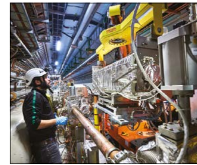
Installation of a collimator at LHC point 1.
