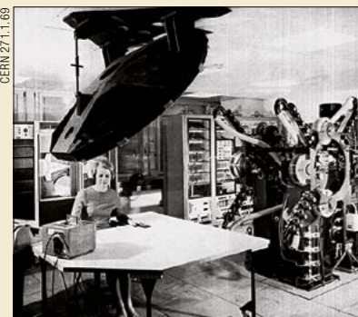
(Top) On 26 February, the Spiral Readers at CERN clocked up their millionth measured event on bubble chamber film. This type of semi-automatic measuring machine was initiated at Berkeley. Two have been built at CERN, the first coming into action for regular film measurement in 1970. They both now operate at a rate of about 70 vertices per hour.
