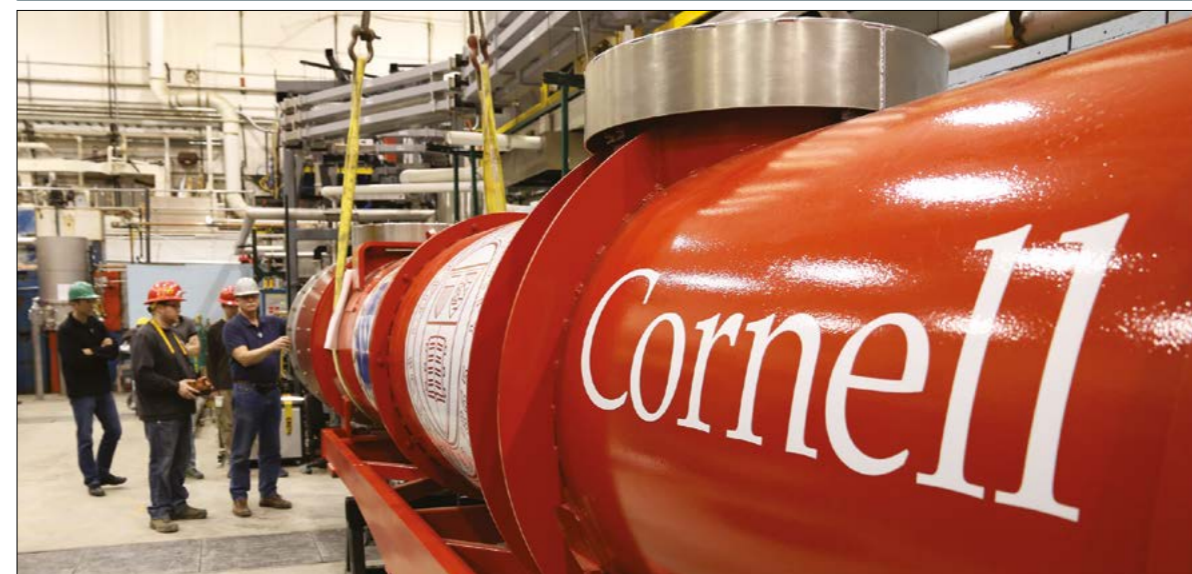
The main linac cryomodule for the Cornell-Brookhaven CBETA facility being moved into place in February 2017.
