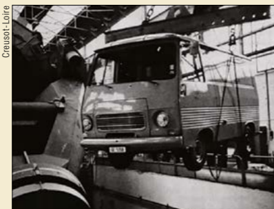
The van being lowered into the pit, where the 3.6 m ESO telescope is installed, plays an important part in the tests now underway. It is a mini-electronics laboratory for controlling the telescope operation, equipped by the ESO unit working at CERN.
